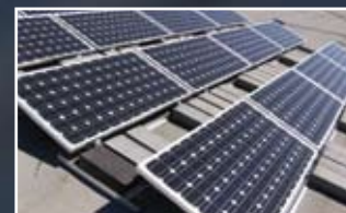
FLAT ROOF BALLAST SOLUTION
